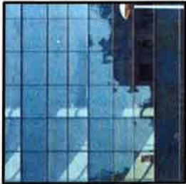
GREY TINTED LOW-E GLASS TO TOWER FACADE
